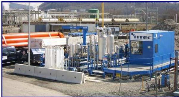
Figure 1. Hydrogen capture, purification and compression plant.
