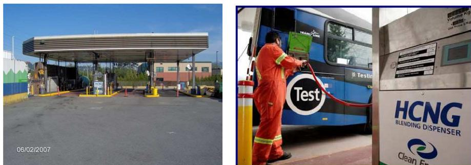
Figure 3. Refueling of a HCNG bus at the Port Coquitlam HCNG station.
