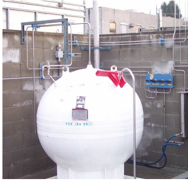
Figure 4. HCNG fuel mixing and storage.
