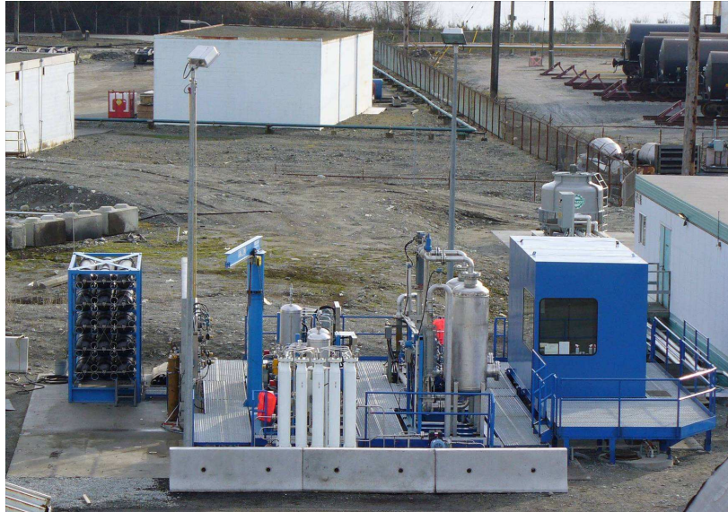
Figure 2. Hydrogen capture, purification and compression plant.
